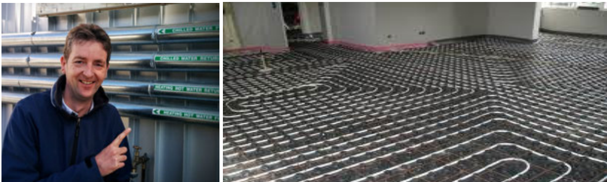
Thermal energy distribution with closed loops of water, in the floors and walls
